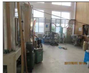
Photo of the inside of the main production hall Mixing workshop.JPG
