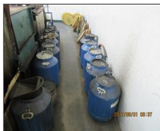
Photo of non-conformity No secondary containment and MSDS.JPG
